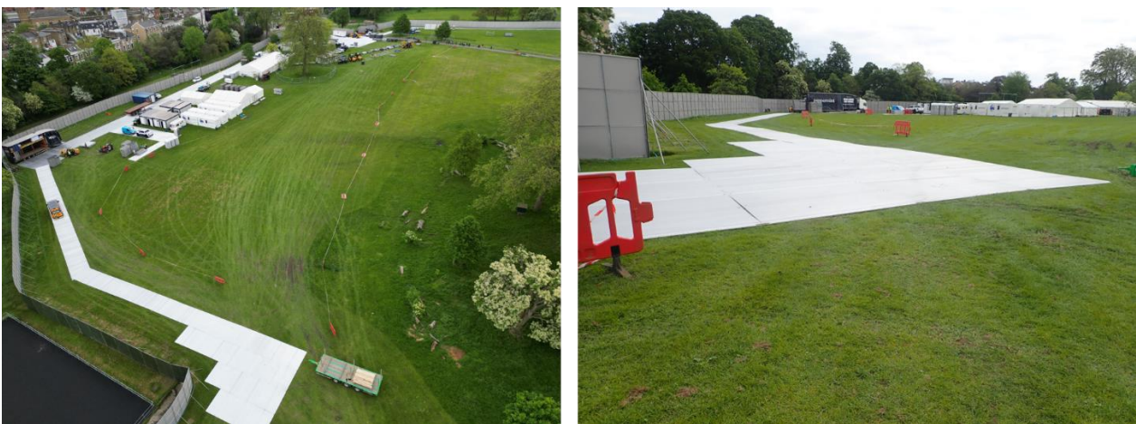
Figure 1-2 Trackway, installations and fencing being installed in Red Gate area
