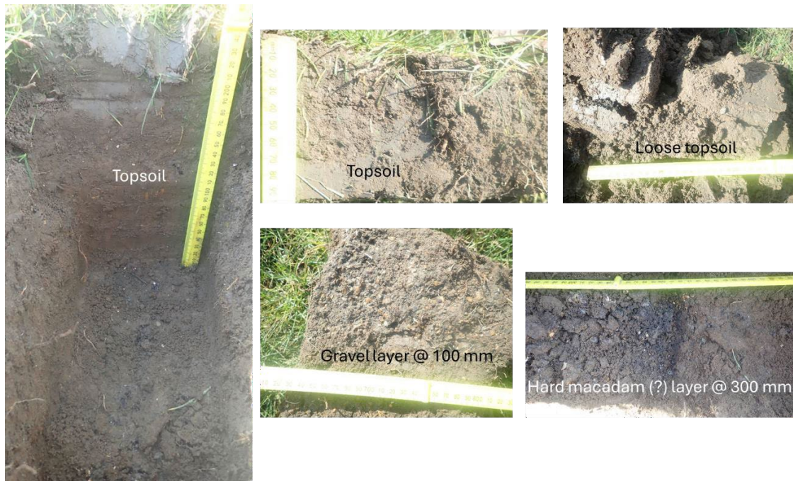
Figure 3-2 Features of the soil profile of the entrance area
