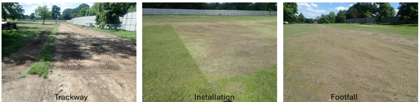
Figure 2-6 Examples of damage types
